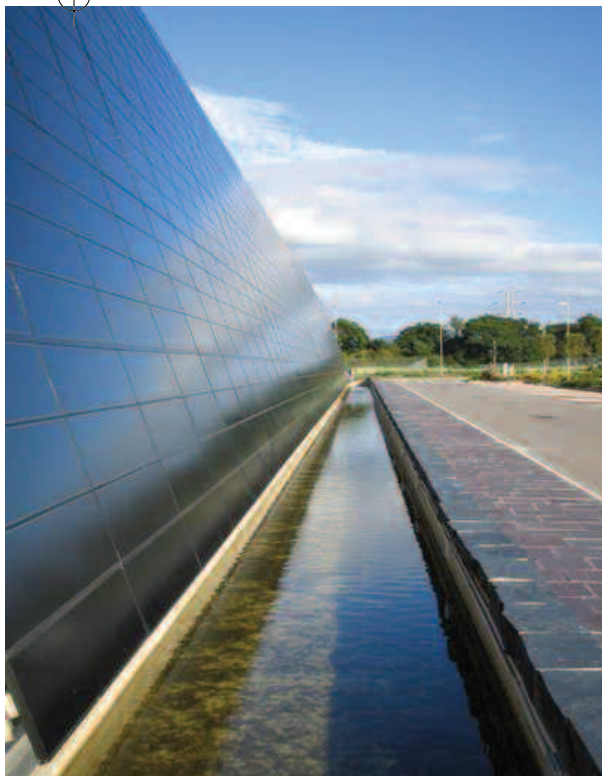
Technium at St. Asaph: helping to develop new Welsh ideas
