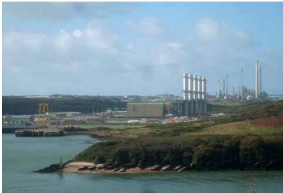
When it is up and running the new Pembroke power station will extract 3,456,000 cubic metres of water from the Milford Haven waterway each day – equivalent to three times the combined flow of the two Cleddau rivers.
