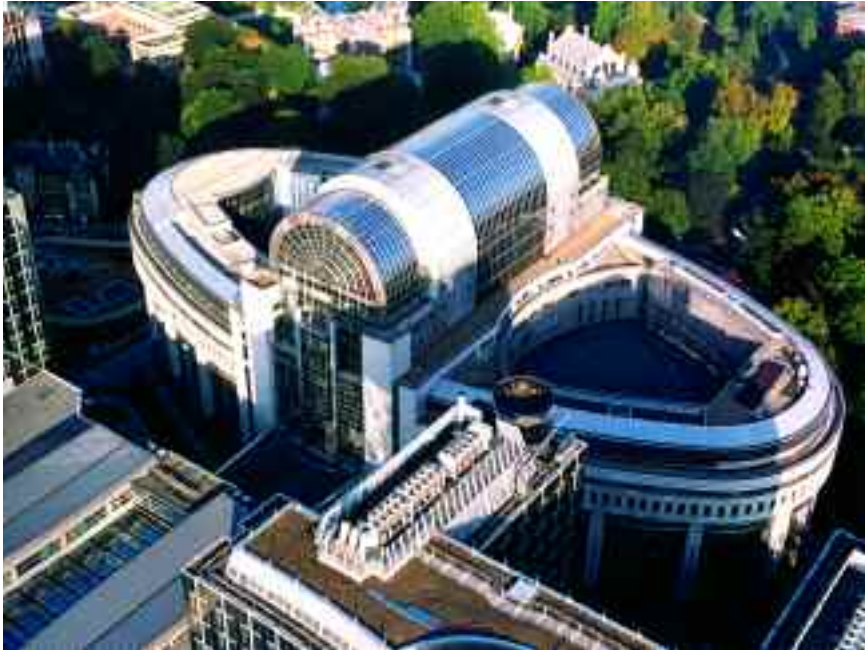
Dwarfing all other political building in the world – the European Parliament in Brussels.
